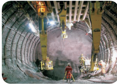
Vortrieb Einspurtunnel Ost Nord Excavation of single line tunnel East North
